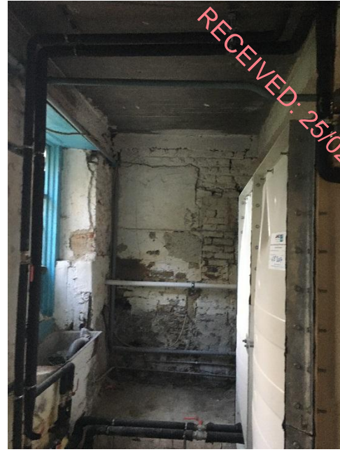
Fig. 34 View east in same room
