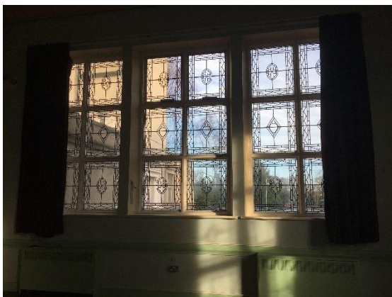
Fig. 50 North elevation leaded window
