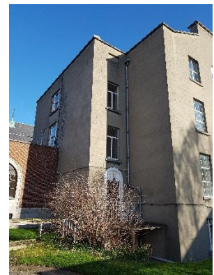
Fig. 38 The original extension rear wing to west, matching the southern (extended) gable of Milltown Park House
