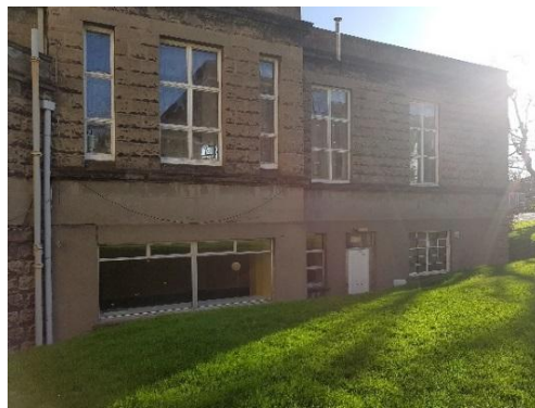
Fig. 47 View of west elevation
