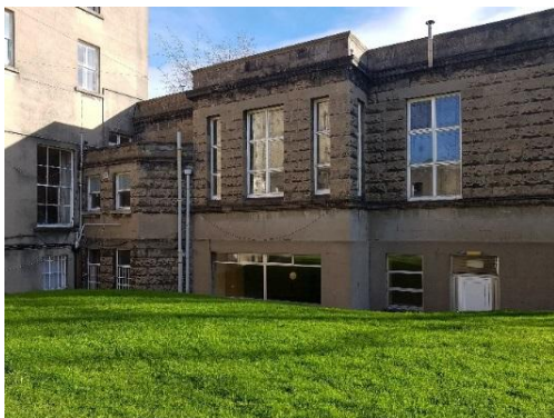
Fig. 46 View of west elevation
