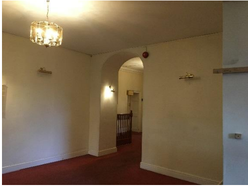
Fig. 29 Infilled entrance hall at entry level with modest access to rear inner hall, leading to the late 19 th century extension block. Stair visible through the arch accessing upper floors.
