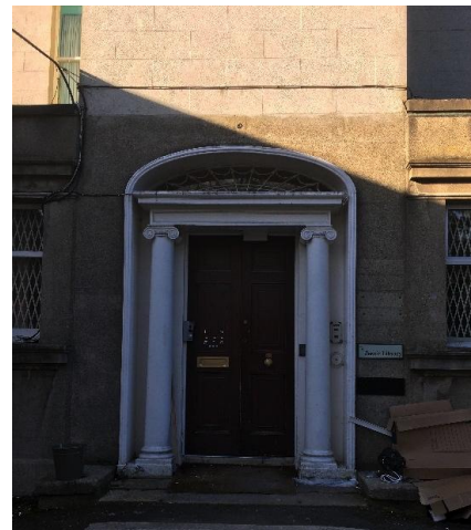
Fig. 22 Detail of the surviving entrance door and fanlight within a much-altered context.
