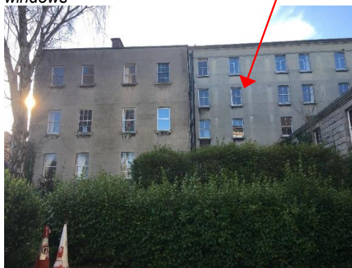
Fig. 23 North elevation of Milltown Park, which was vertically extended in the late 19 th century. The north elevation of its rear, higher, extension was constructed in the 20 th century.
