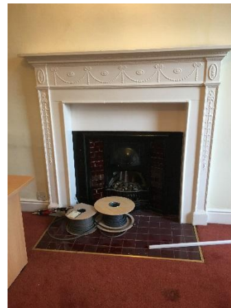
Fig. 32 Early chimney piece with later tiled inset and hearth, in same room.
