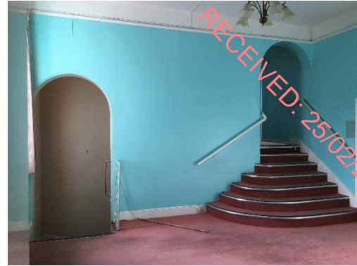
Fig. 30 First floor level infilled entrance hall with later wall painted blue. Curved stair leads to vertical extension wing above a former orangerie.
