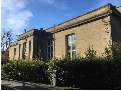
Fig. 43 View of east elevation
