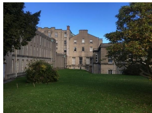
Fig. 24 Southern elevation, comprising an extension, with its expressed gable. Note the uncomfortable connection with its rear, later, extension, at a storey higher.
