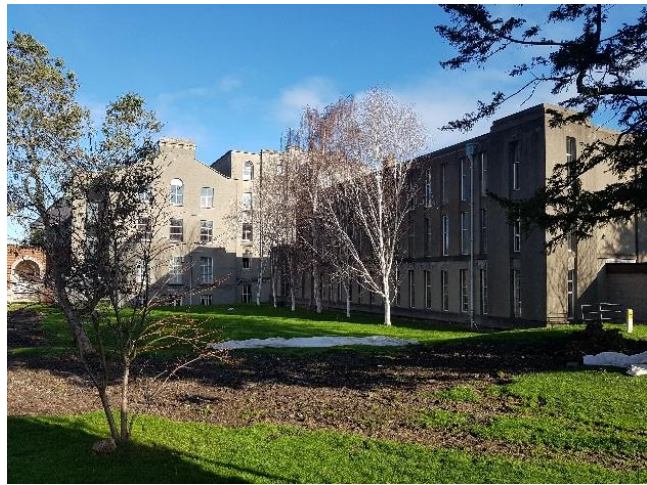
Fig. 56 West elevation in context with Extension Block
