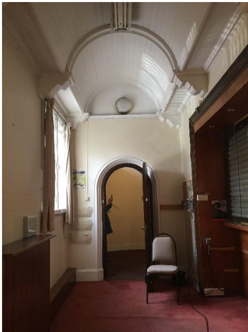
Fig. 27 Entrance vestibule, towards the entrance porch
