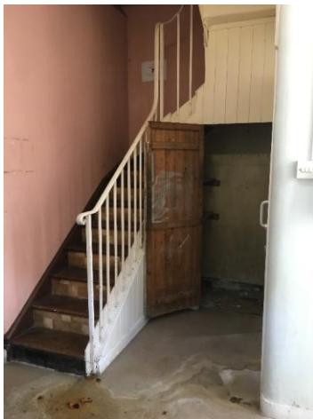
Fig. 70 Secondary steel stair of interest
