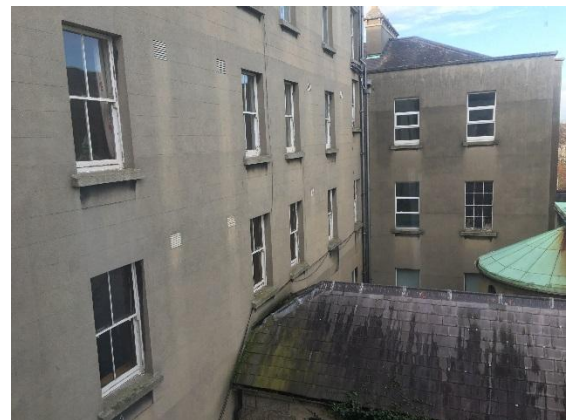
Fig. 40 View of the (later) northern extension from a rear 1 st floor window of Milltown Park house, towards the opposing (original) H form comprising a lower building, possibly intended to align with MPH.
