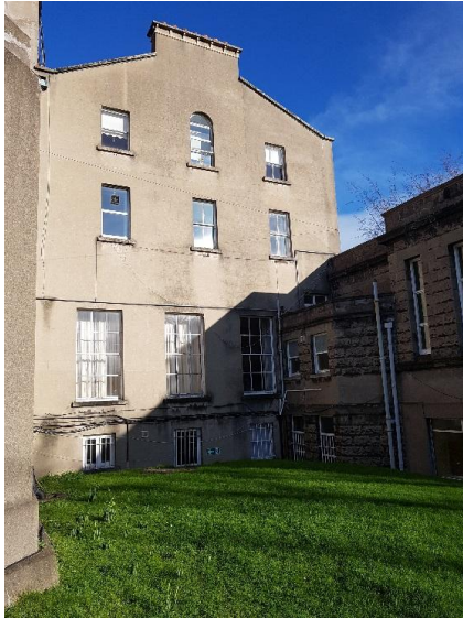
Fig. 25 Southern elevation, comprising an extension, with its expressed gable in context with the Finlay Wing and Archive (corner visible). Lower windows are early in origin, with the 6/6 windows attached to a former orangerie, which was vertically extended in the 20 th century.
