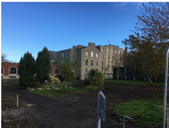
Fig. 39 Southwest view of the original extension, culminated in an expressed H form gable building corresponding with an addition to the main house, (F.21 above). The taller central section is a later addition.
