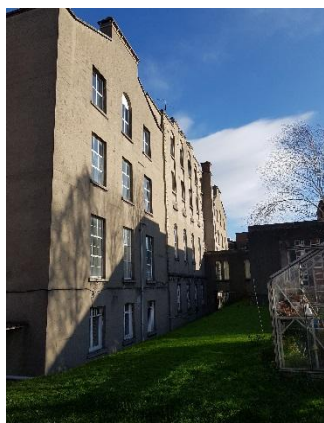
Fig. 41 View from west
